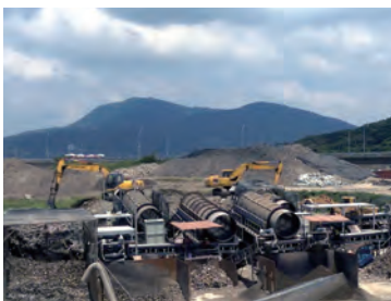
Taipei Port Resident Recreation Area Waste Removal Project
