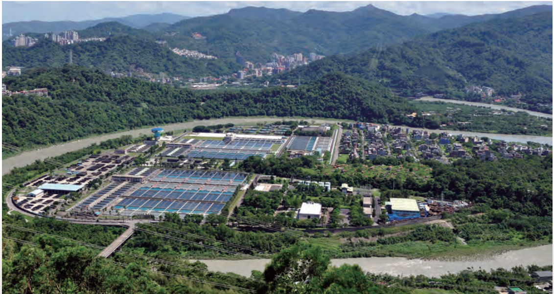
Improvement Construction of First Quick Filter Pool Equipment in Zhihtan Water Treatment Plant, Taipei City
