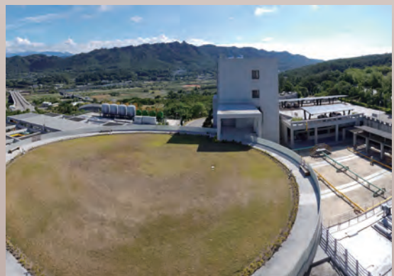
Management of Turnkey Project for Function Enhancement of Conductivity Treatment Facility in Tonglu Wastewater Treatment Plant of Hsinchu Science Park
